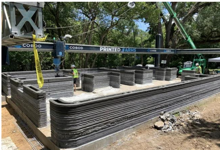
3D Printed house under construction in Tallahassee [Source: Tallahassee Democrat]
