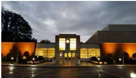
Tiffany & Co. Customer Fulfillment Center, Parsippany, NJ [Source: BusinessYab]
